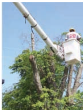
Allen Williams (Light and Power) in bucket
